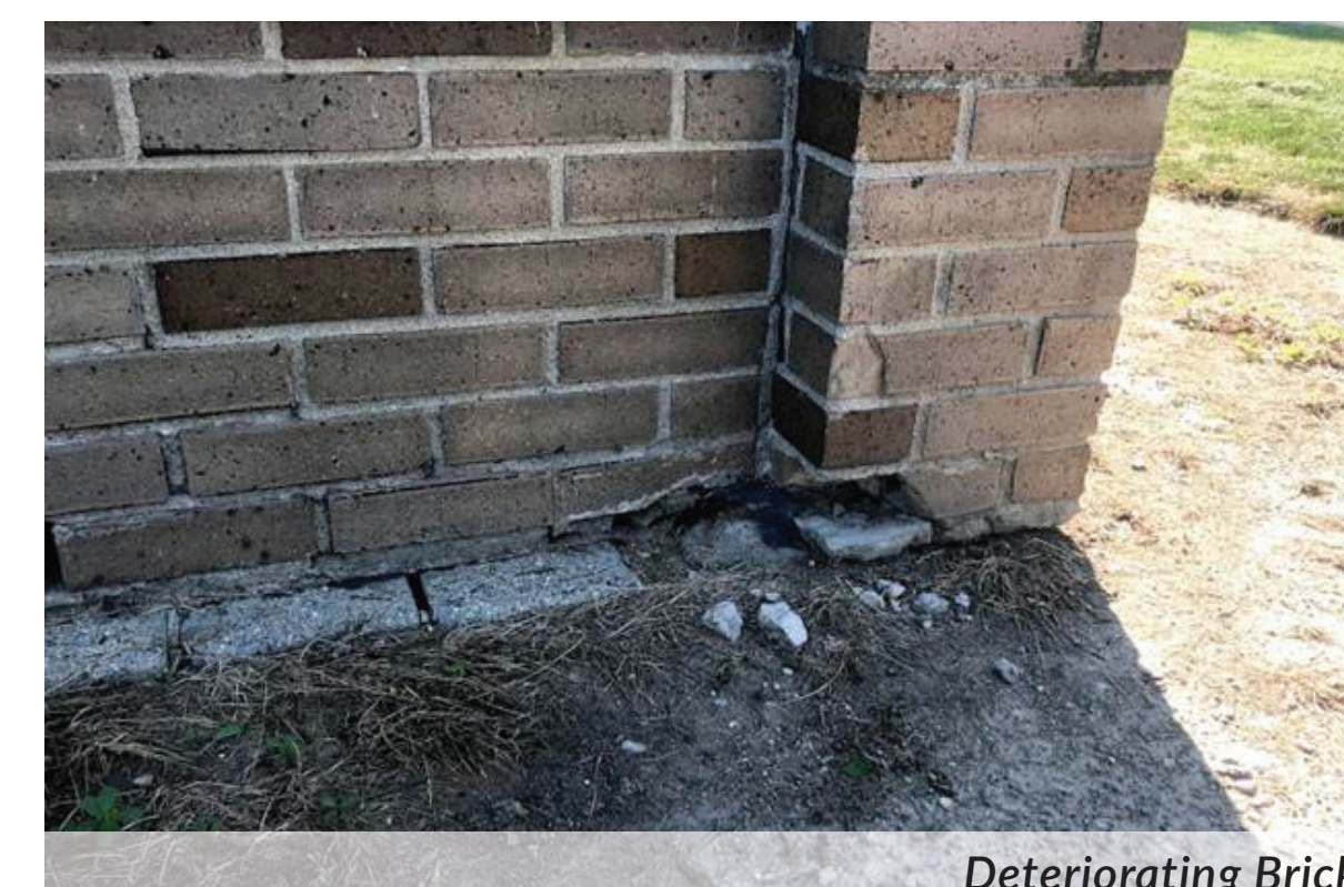
Deteriorating Brick
